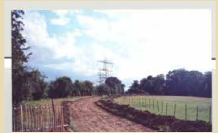
August 1996 (Road Construction)
